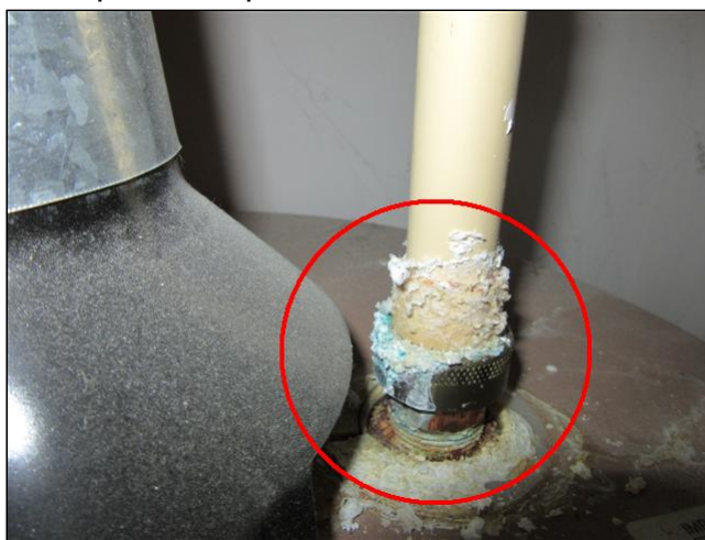
6.1 Item 1(Picture) Corrosion noted at hat water heater plumbing.
