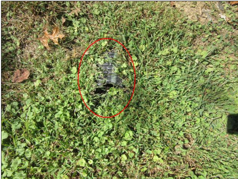
1.3 Item 2(Picture) Buried gutter downspouts should be opened and allow water to flow as intended.
