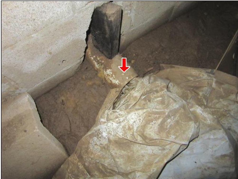
5.0 Item 3(Picture) Drain at crawlspace stopped up.
