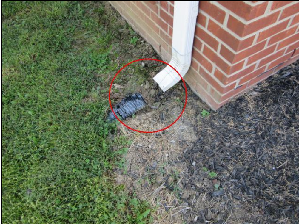
1.3 Item 1(Picture) Downspout disconnected.
