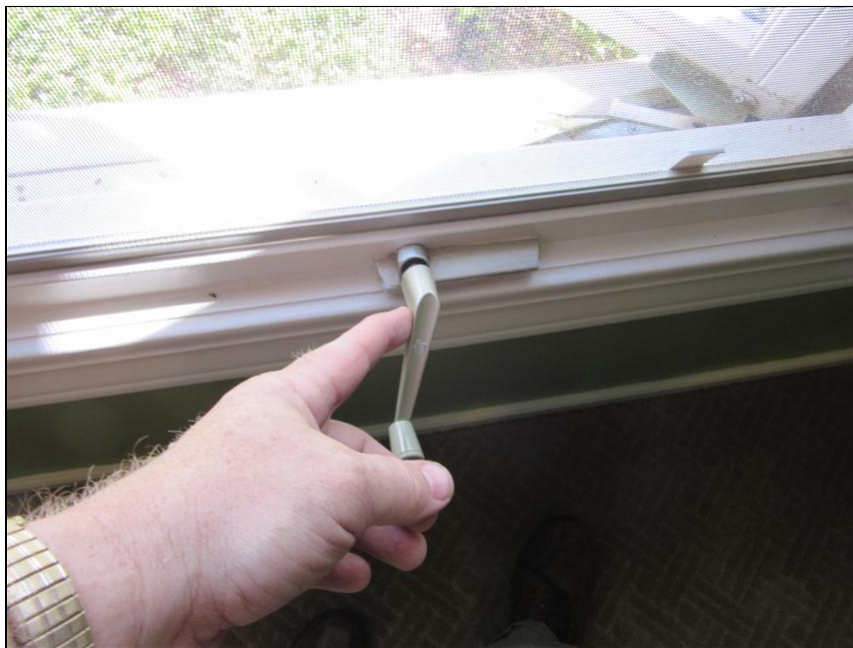
2.2 Item 1(Picture) Damaged window opening mechanism.
