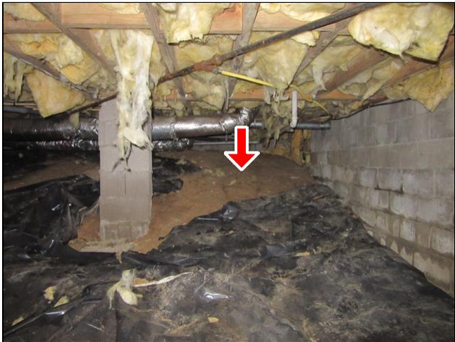
9.2 Item 1(Picture) Vapor barrier missing at places.
