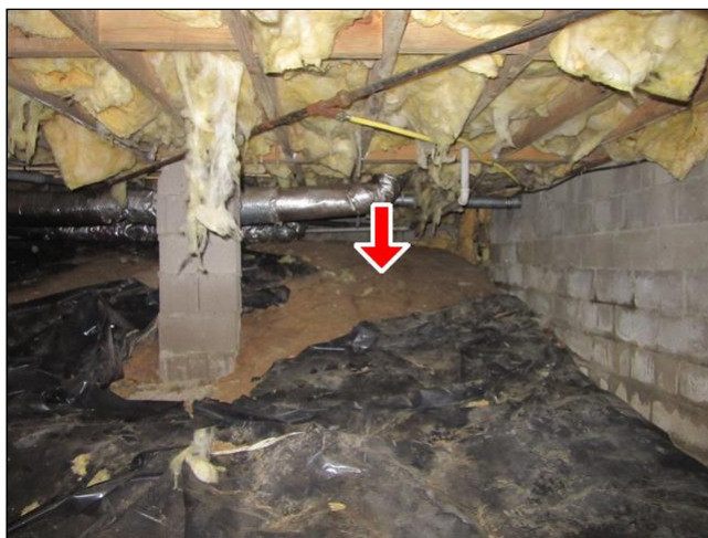
9.2 Item 1(Picture) Vapor barrier missing at places.
