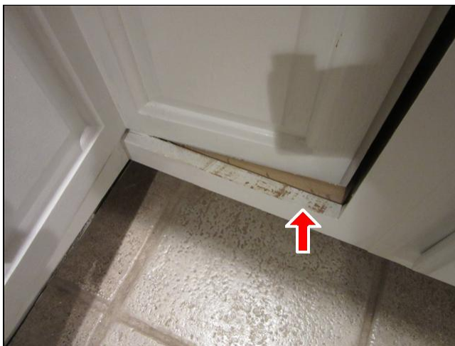
4.4 Item 1(Picture) Lazy susan door rubbing at bottom.
