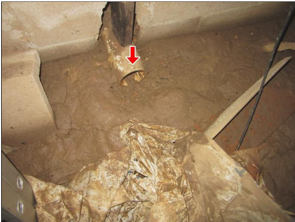
5.0 Item 4(Picture) Same drain after removing debris.
