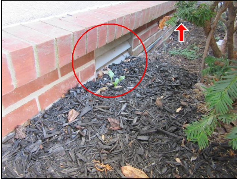
9.3 Item 1(Picture) Two foundation vents are below grade.
