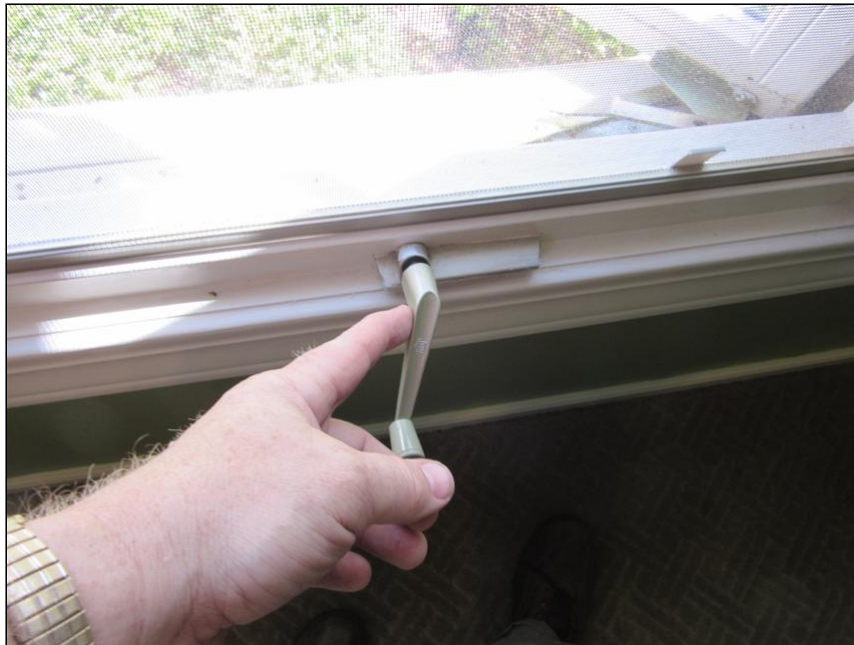
2.2 Item 1(Picture) Damaged window opening mechanism.
