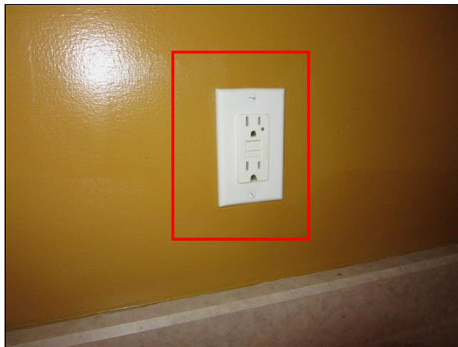
7.5 Item 1(Picture) GFCI type receptacle would not trip when tested.(kitchen)
