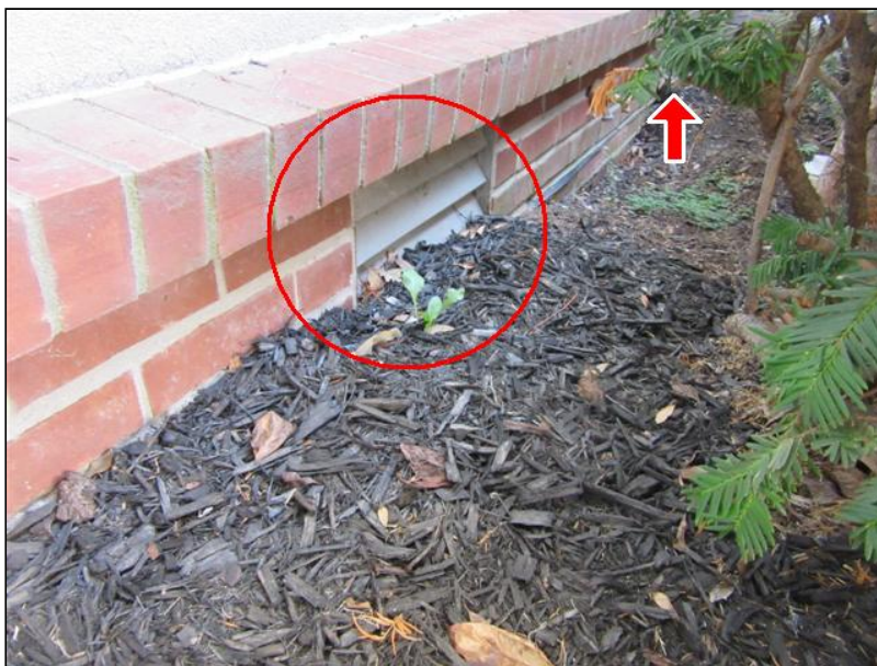
9.3 Item 1(Picture) Two foundation vents are below grade.
