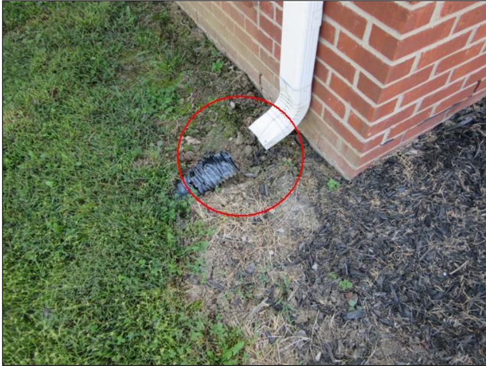
1.3 Item 1(Picture) Downspout disconnected.
