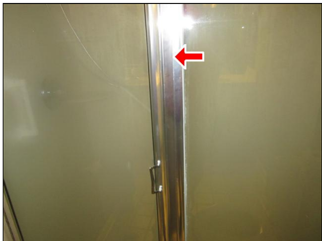
4.5 Item 1(Picture) Shower door rubbing when operated.
