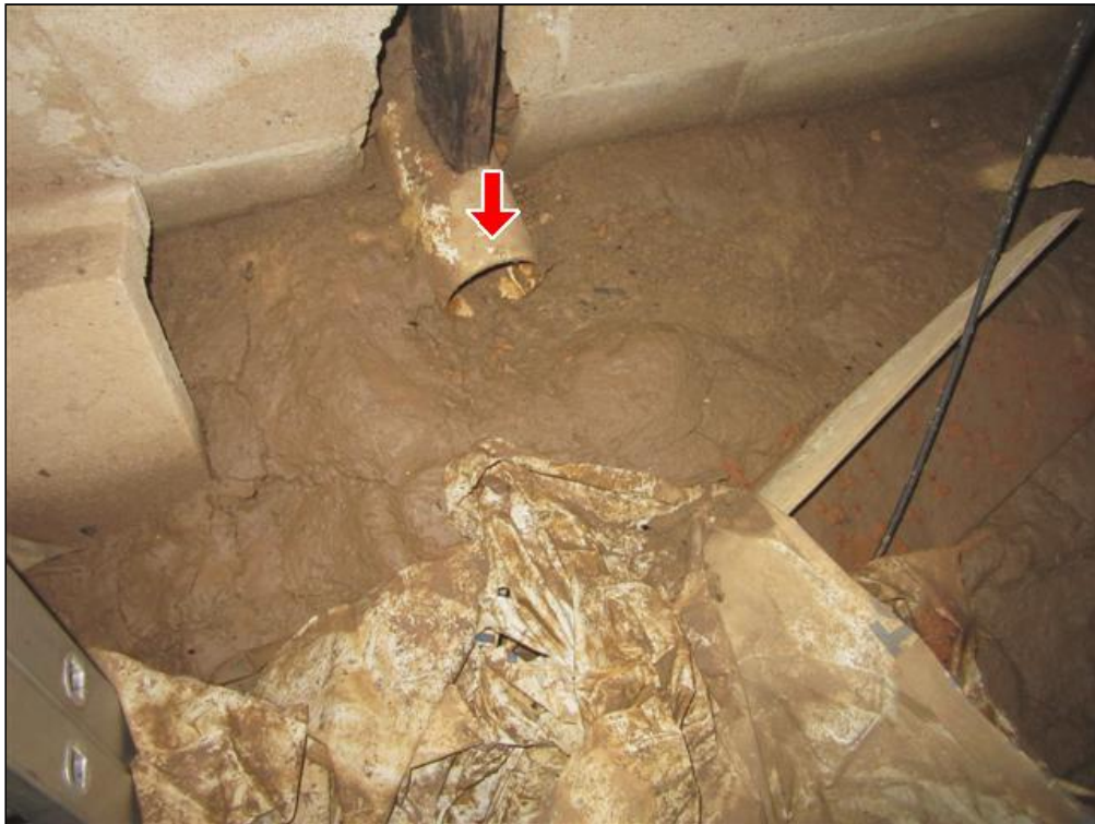
5.0 Item 4(Picture) Same drain after removing debris.
