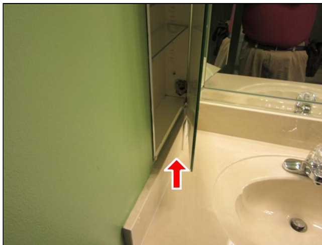
4.5 Item 2(Picture) Medicine cabinet door does not close properly.
