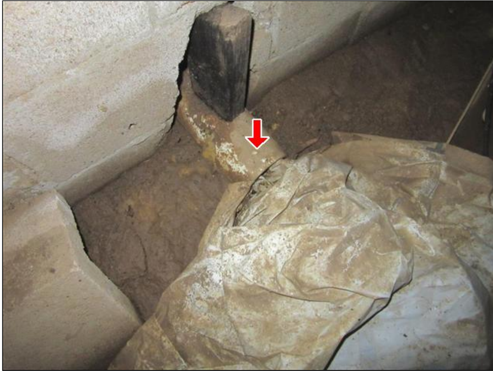
5.0 Item 3(Picture) Drain at crawlspace stopped up.
