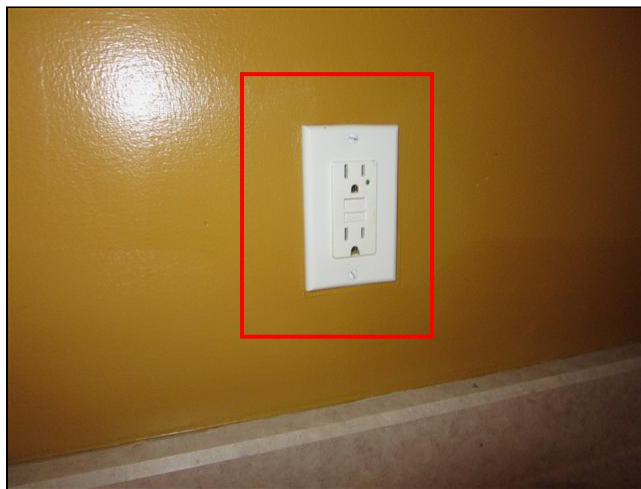
7.5 Item 1(Picture) GFCI type receptacle would not trip when tested.(kitchen)
