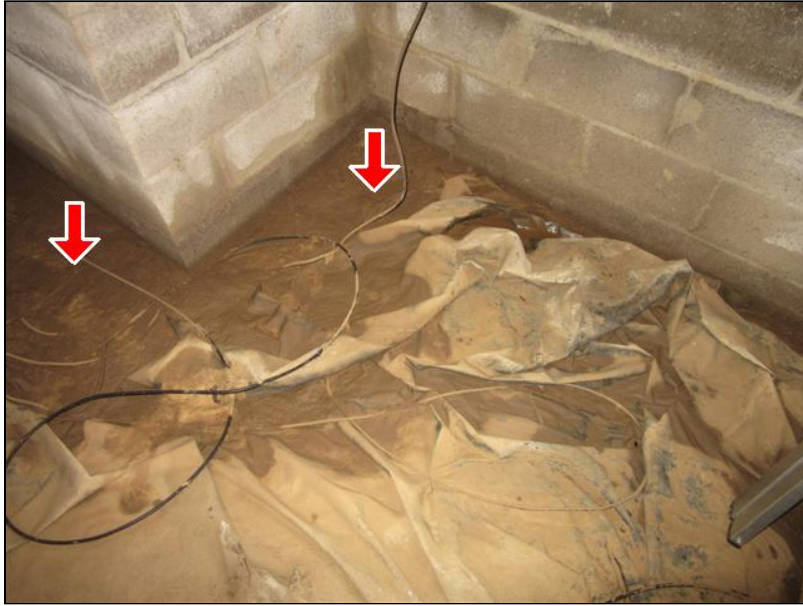
5.0 Item 1(Picture) Some standing water noted at crawlspace.
