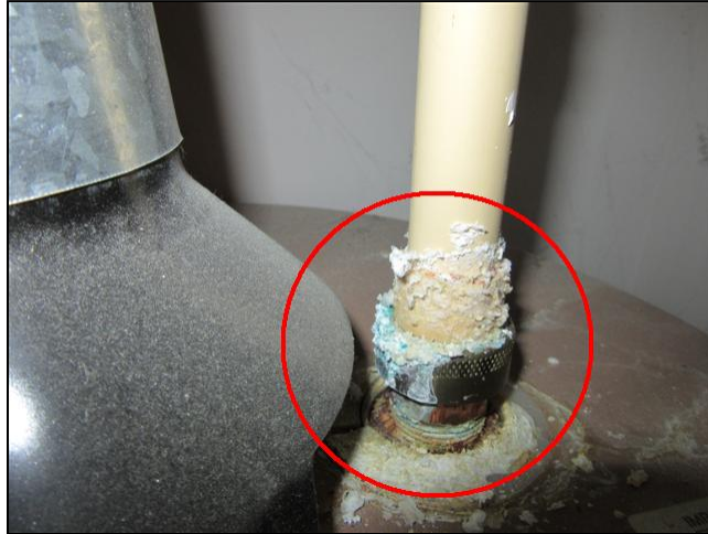
6.1 Item 1(Picture) Corrosion noted at hot water heater plumbing.
