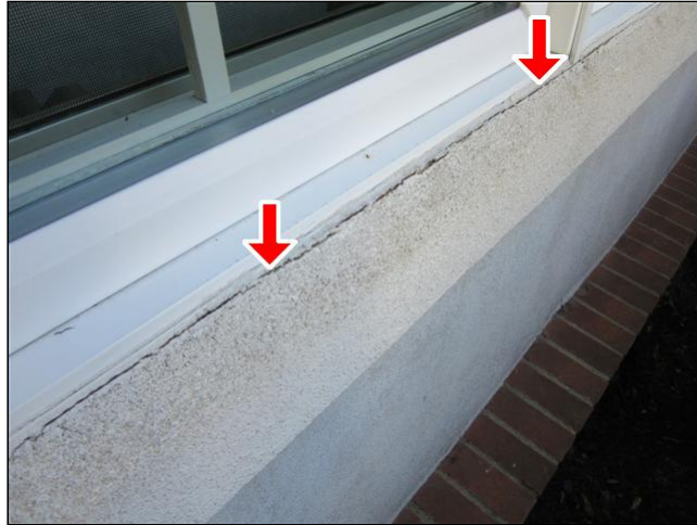
2.0 Item 1(Picture) Maintaining caulk at exterior with this type of exterior finish is critical.
